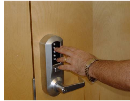
Figure 3-11. Cipher Lock System
